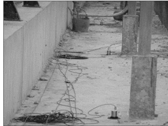
Fig 8: Picture showing vertical accelerometers mounted on the bridge deck
